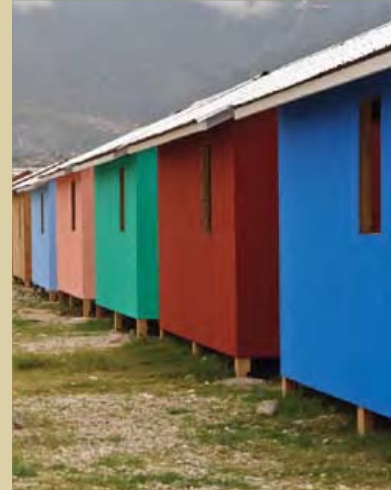
Completed Red Cross transitional homes in La Piste, Port-au-Prince.
